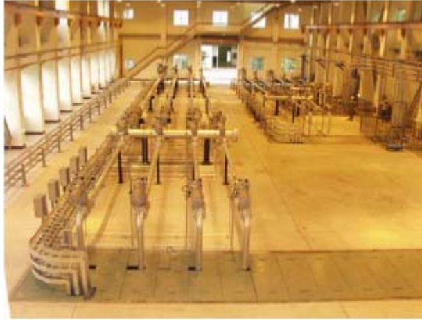
CPC High Pressure Air Flow Facility
